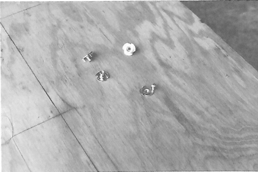
Tee nuts should be secured with small screw before covering.
